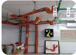
Plumbing and electrical piping construction method demonstration
