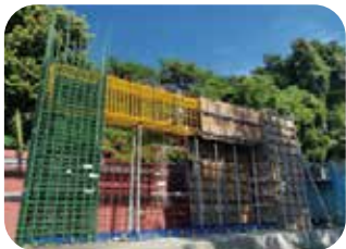
Steel reinforcement construction method demonstration
