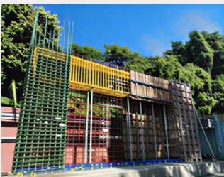
鋼筋工法示範
