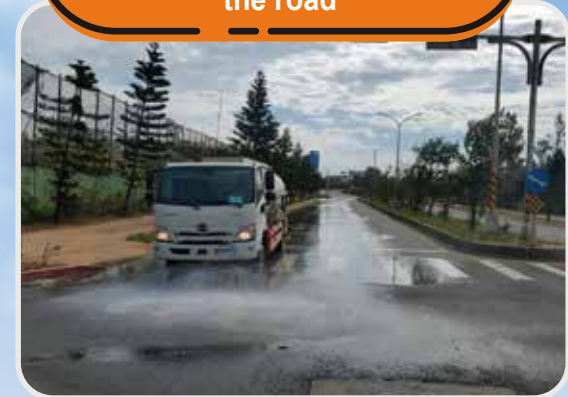
Water spraying for dust suppression near the road
